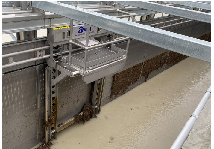
Above: The flat-screen cleaner dealing with a heavy workload during the 19 July 2022 floods.
