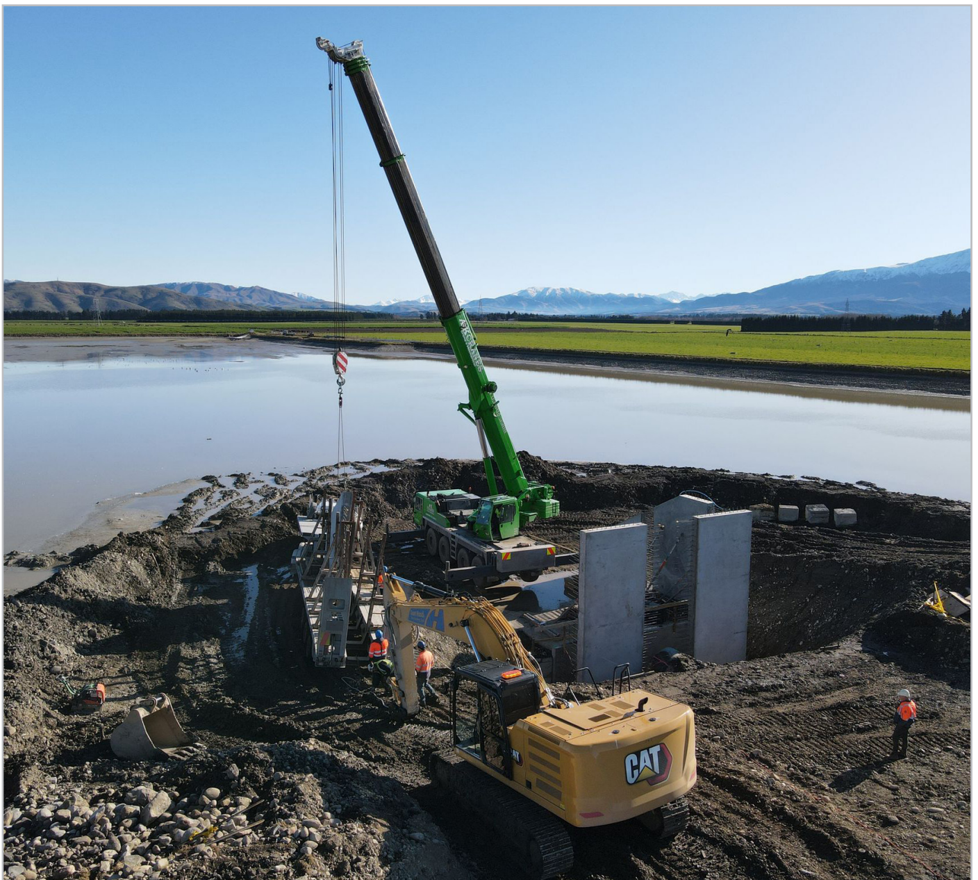
Concrete panels being craned into place for the concrete structure that will support the Andar screens.
