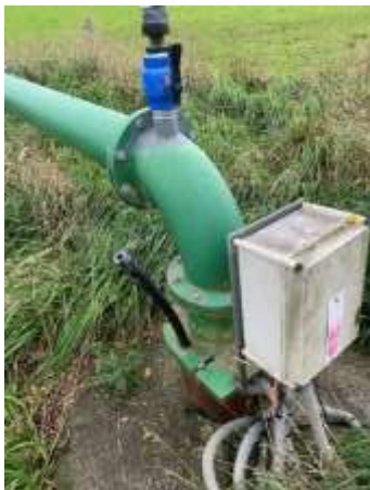
Figure 74 Well head with alkathene conduit
