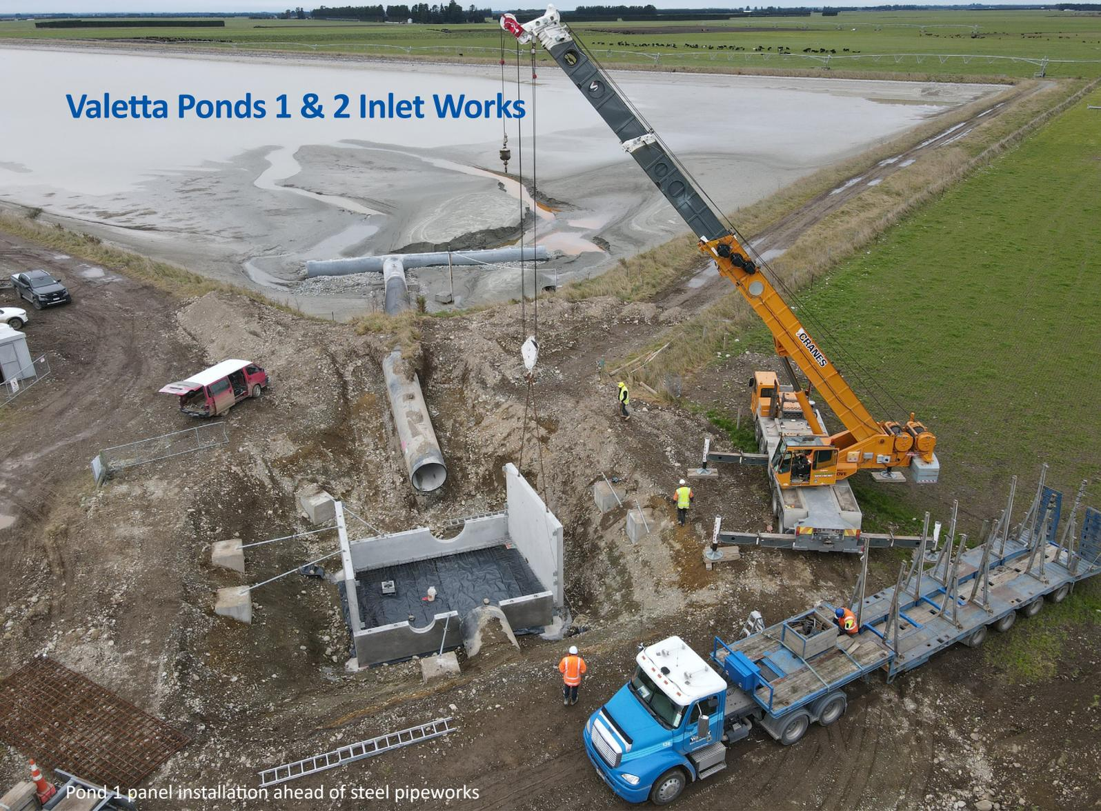
Work is well underway on the winter workstreams to upgrade Valetta Ponds 1 & 2 inlet infrastructure. The work is being undertaken to address asset and operational risks identified in the Valetta Masterplan.
