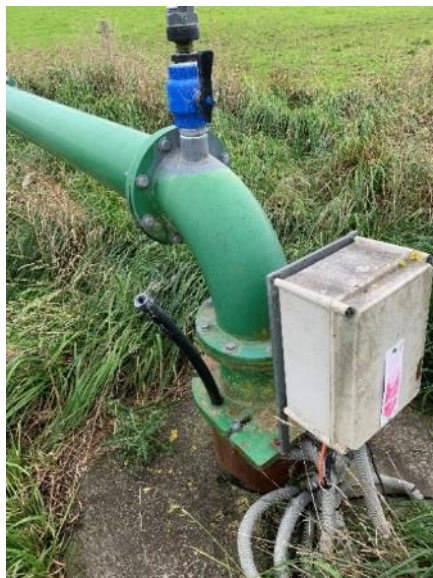
Figure 26 Well head with alkathene conduit
