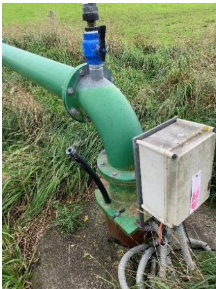
Figure 26 Well head with alkathene conduit
